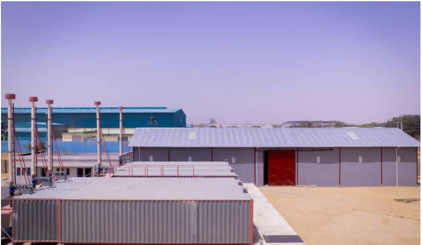
Sourcing and Produce's new warehouse and fumigation chambers.
